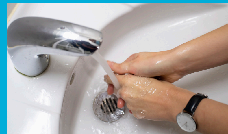
Sensor taps in restrooms (Photo: Lars Horn, Baghuset)
